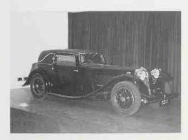
S.S. 1 coupe in its final form. The full front fenders flow into running boards. The proportions of the hood, roof and doors have been adjusted so that the edge of the hood, the bottom of the side window lines and the lower edge of the fabric covered roof all line up. Windshield wipers have exterior linkage.
